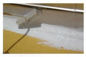
Usage of reinforcement is recommended, especially over floor & wall joints and areas of expansion. Use fiber glass reinforcement mat embedded into first coat while still wet. Press and smooth with roller. Apply the second coat, as mentioned above.
