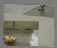
4. Dampen the surface thoroughly with water and apply the mixed material using a soft bristled brush/roller/ trowel, in two coats, to acheive
