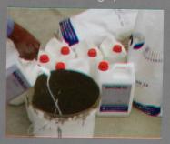
Pour the liquid polymer component in to the mixing drum.
