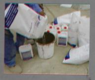
3. Add the powder component to the liquid. Stir thoroughly for 3-5 minutes until the mix is homogenous & lump free, using a paddle attached to slow speed drill.
